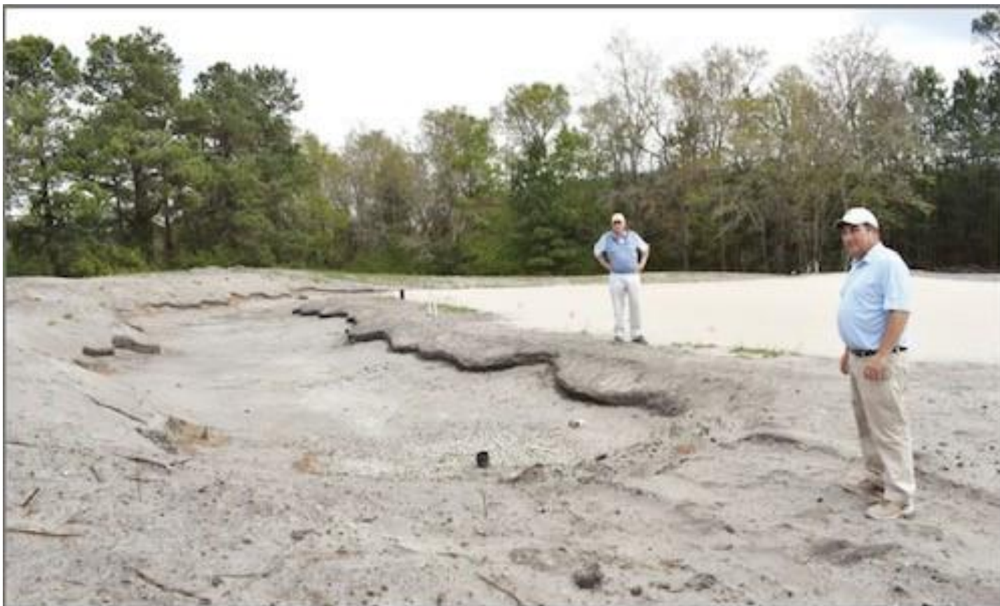
Scalloped bunkering is one of the features of the new design at the Wellman Club, produced by Rees Jones and Bryce Swanson.
